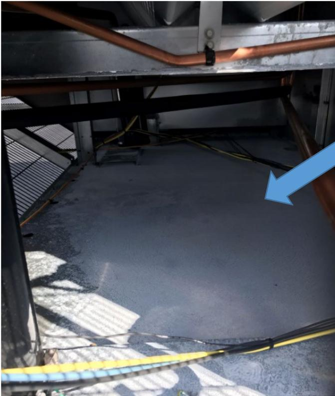
Minimizing moisture build up can help in minimizing WSS, but in most cases, it can't be avoided. WSS will not impact the service life of HVAC equipment nor will it impact the warranty of the product.
